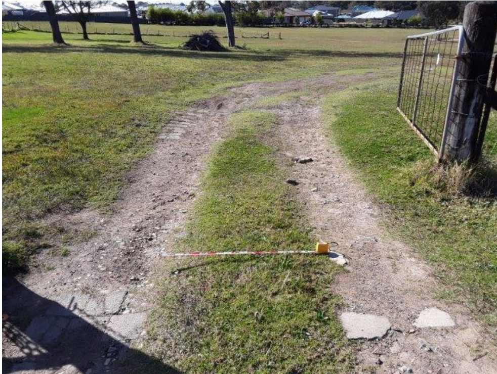
Photo 13 Exposure within vehicle track
