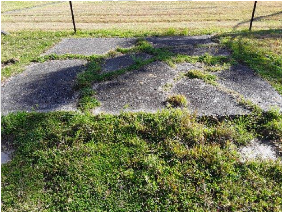
Photo 17 Concrete slab within the central portion of the study area
