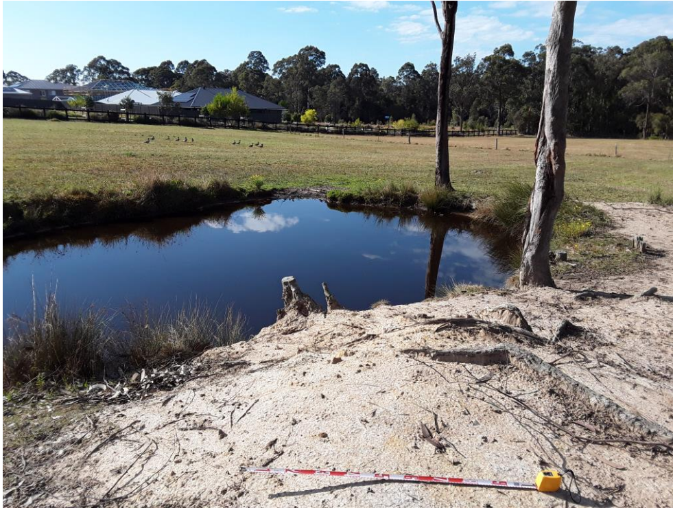
Photo 15 Area of exposure under trees adjacent to dam
